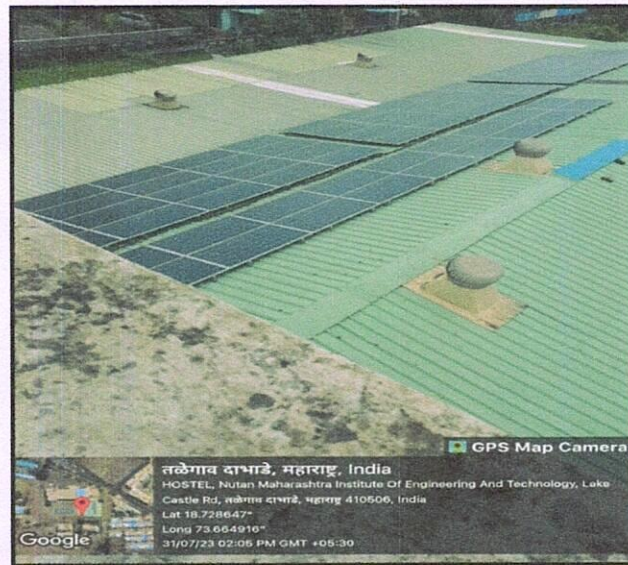
Photograph of Roof Top Solar PV Plant:
