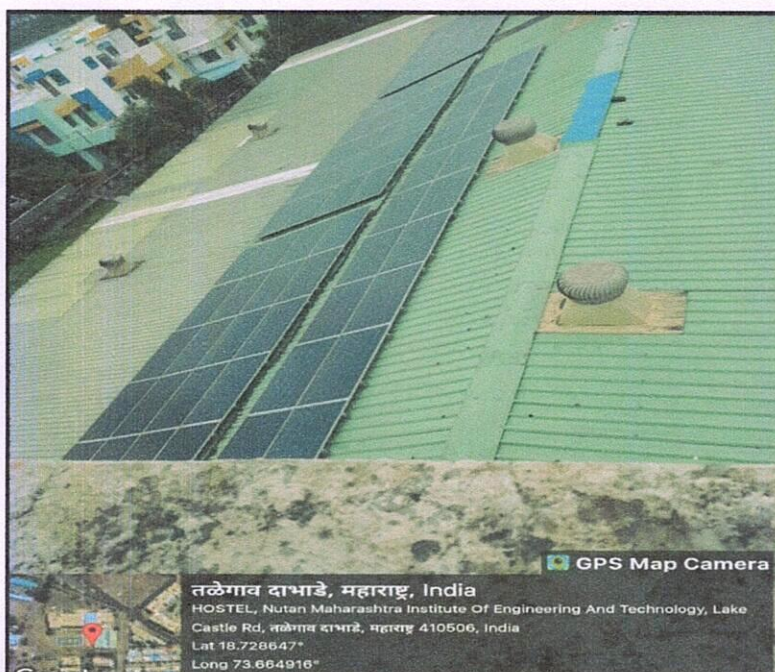
Photograph of Roof Top Solar PV Plant:
