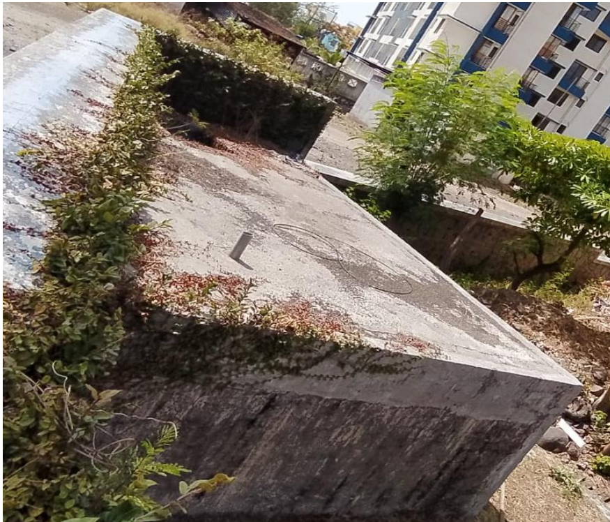
Rain water Storage Tank Annexure 3
